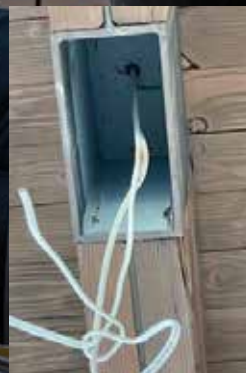
Existing steel boxes – part of the ceiling's exposed beams
